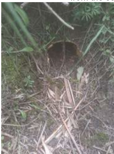
Figure 3. c.5” twin wall plastic field drain
