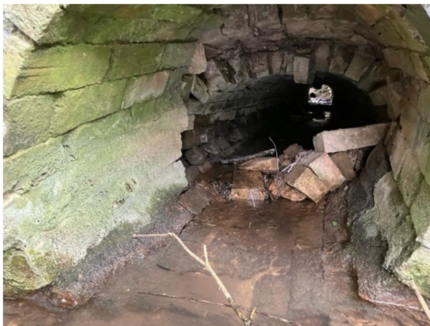
Figure 4. Victorian brick arch culvert
