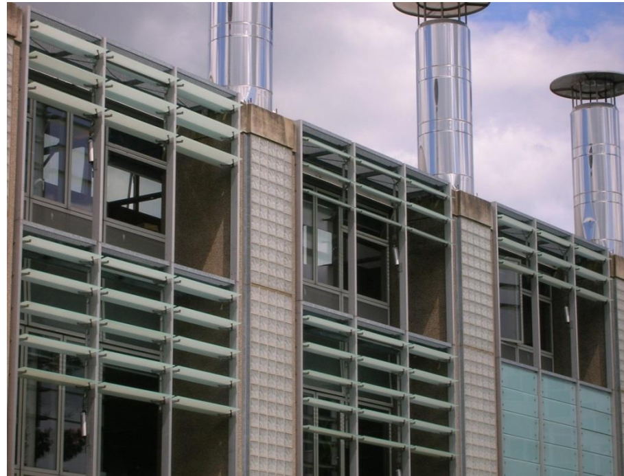
Brise soleil can be used to provide shading and minimise internal overheating. Natural stack ventilation is provided with vertical chimneys.
