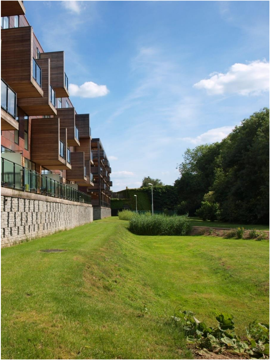
Swales can be used as part of a sustainable urban drainage strategy (SUDs) to attenuate run-off during intense rainfall.
